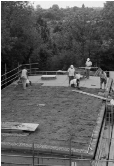
Green roof under construction at Park Lane Nursery, Wembley
